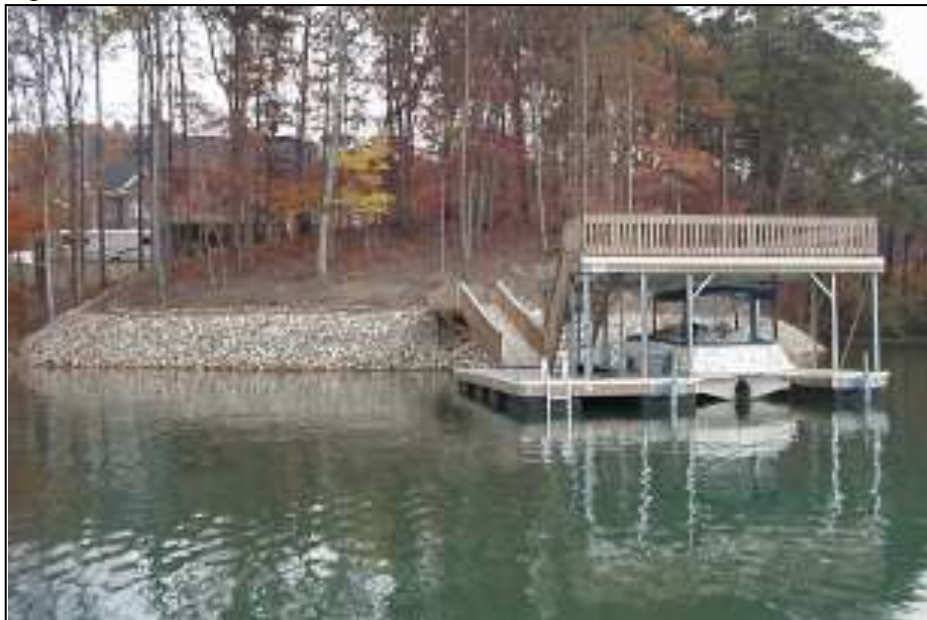
Figure 4: Boat Slip on Mountain Island Lake
